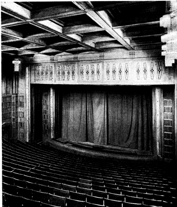
The Künstlertheater, Munich, in which the seating was designed with a constant rise of steps from front to rear. Architect, Max Littmann; 1908
